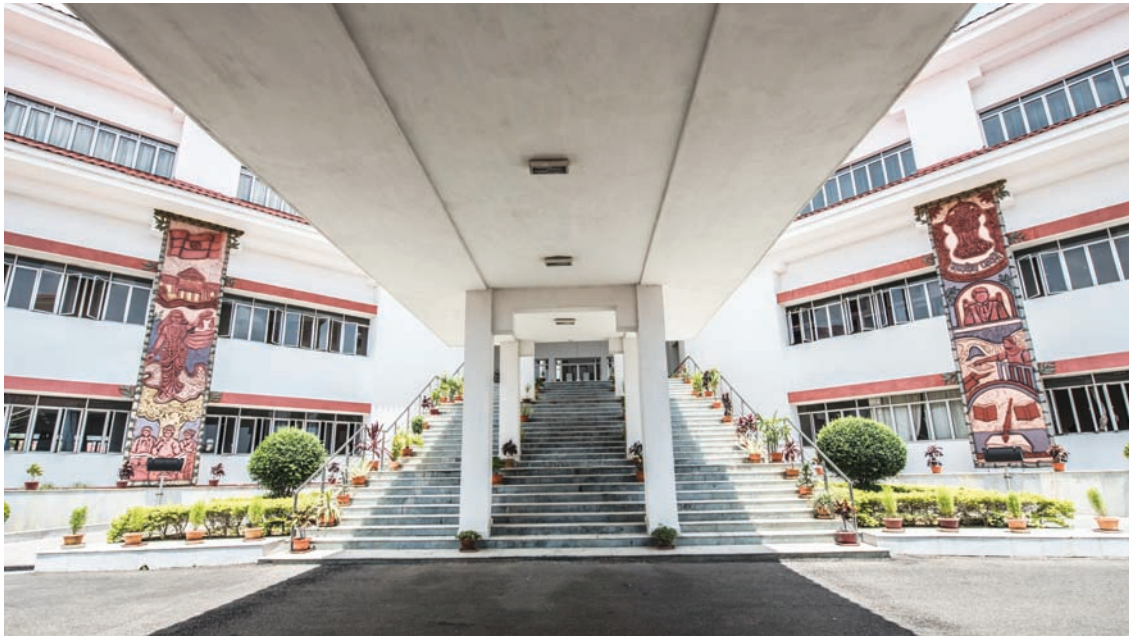
Entrance of the High Court
